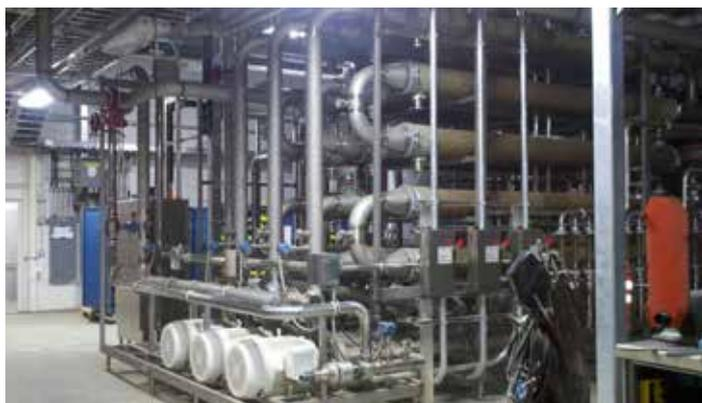
**Picture 1. External AnMBR system with Berghof Membranes UF modules**
