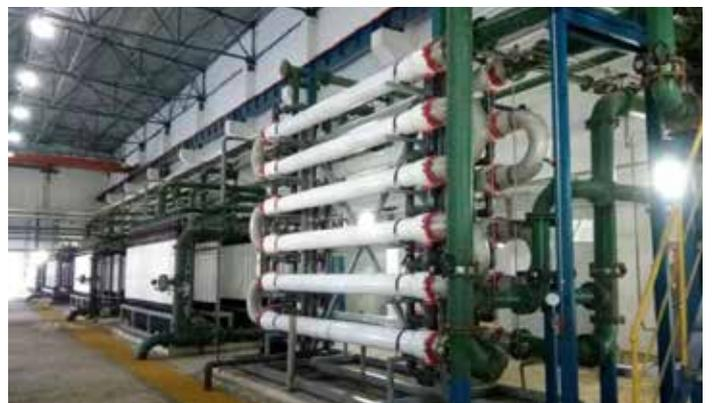
Picture 1. Setup of the tubular UF membranes
