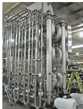
Figure 1: UF system based on Berghof Membranes in Grassland facility.
